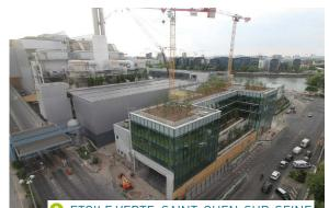
ETOILE VERTE, SAINT-OUEN-SUR-SEINE • Energy recovery unit Catchment area: 1.4 million inhabitants 509,661 tonnes incinerated in 2021 Authorised capacity: 650,000 tonnes Operator: Tiru (Paprec Group)
