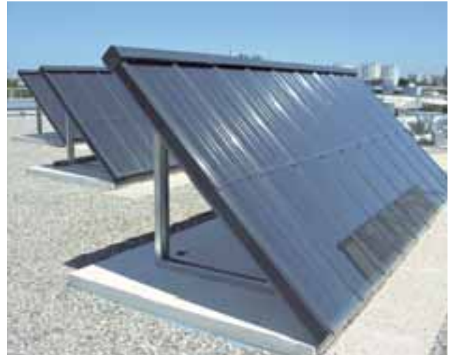
Solar panels installed on the roof of the sorting centre at Nanterre provide for half the needs for domestic hot water.
